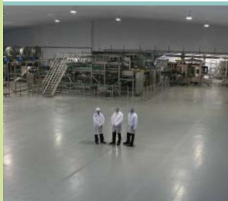
The company furnished its new canning plant with all new equipment, including three PLC controlled retort cookers.
