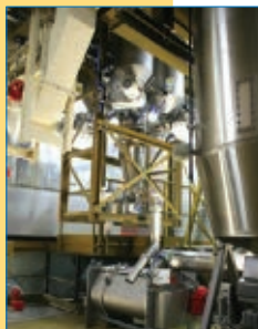
Pegasus vacuum coater, dry dye before extruder and fines and lump separation/sieve.
