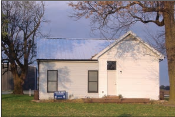
The LEED-certified Novus research facility in St. Louis, Missouri, USA.
