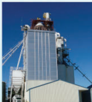
“State of the Art” Conversion, Blending & Packaging Facility.
