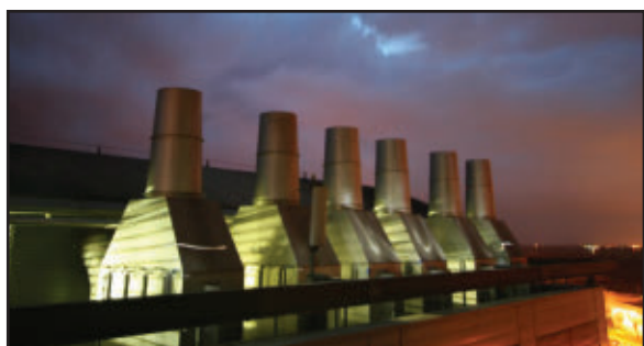
Applied Plasma Physics units provide odor control that meets the high EU regulation standard, according to the company.
