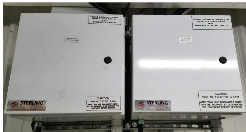
Figure 3: Grinding mill monitors; vibration, temperature tied into automation system
