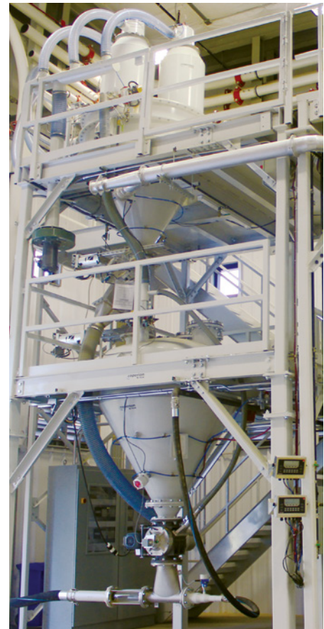
Photo 2 - Dense phase conveying system with rotary valve
