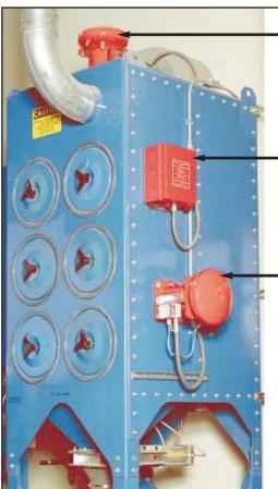
Explosion Suppression Cannon mounted at Dust Collector inlet prevents flames from expanding upstream.
