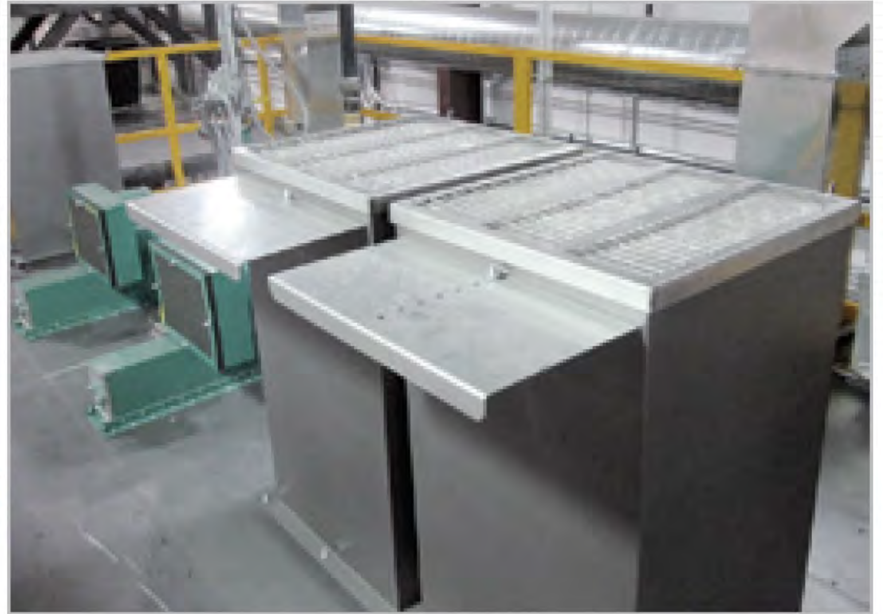
Filtered make up air and burner air to reduce cross-contamination or re-contamination
